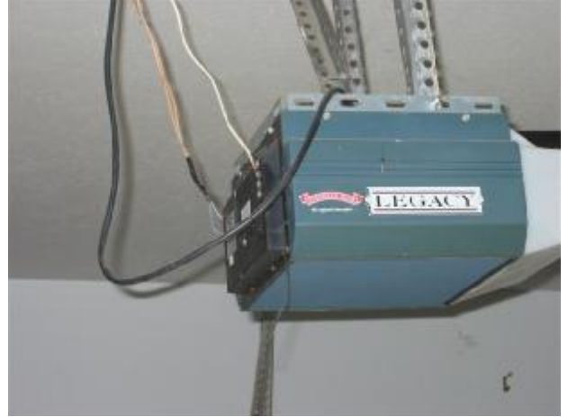
Garage & Carport # GC2
