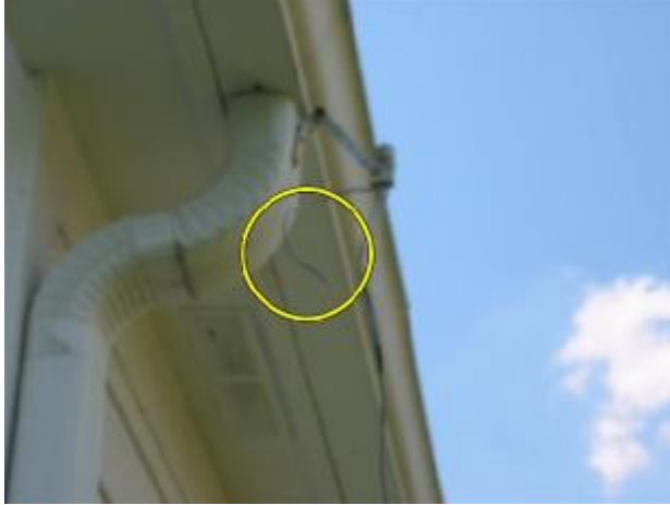
Wiring should be fastened to downspout to prevent it from being torn loose
